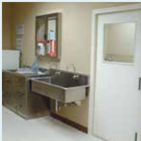
The window finished out with dry wall.
